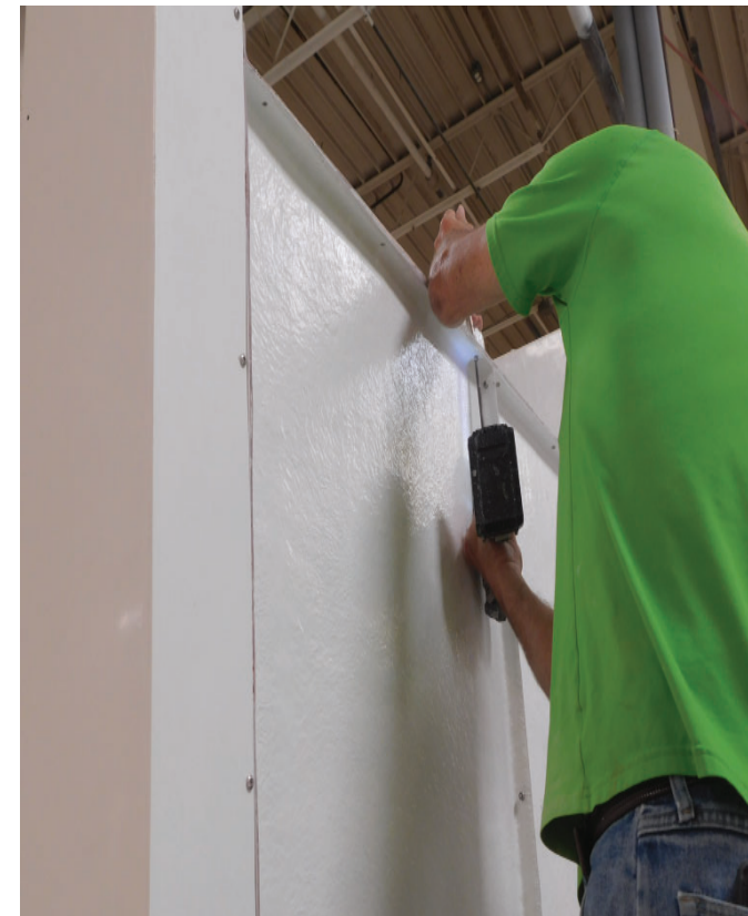
Secure Ceiling Panel to Side Shells with provided #8 or #10 sheet metal screws.
