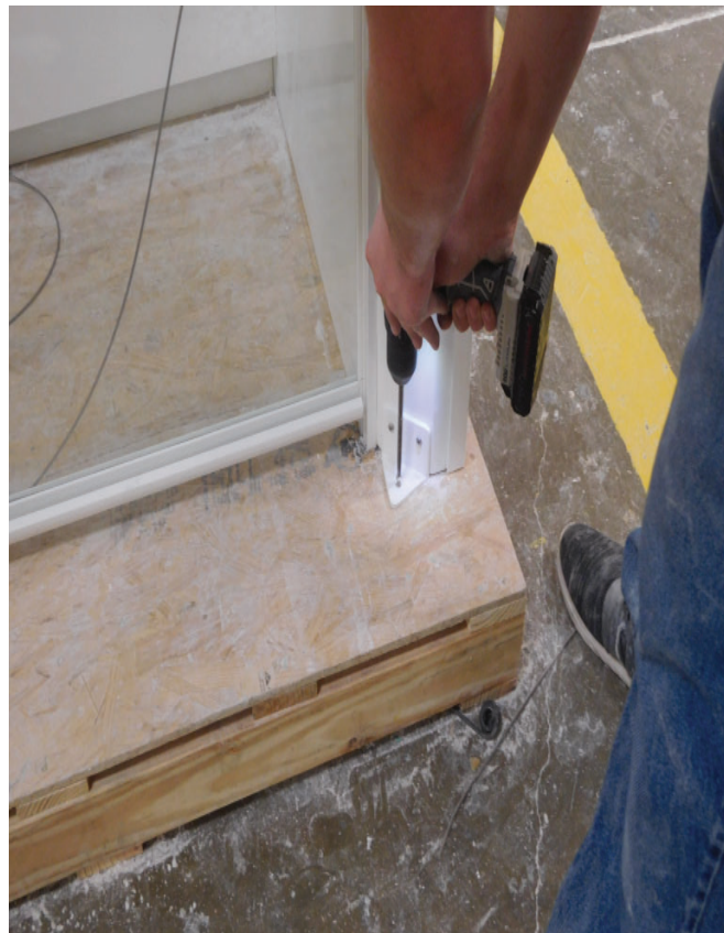
Secure the Front side walls to existing floor with a fastener suitable for floor material.
