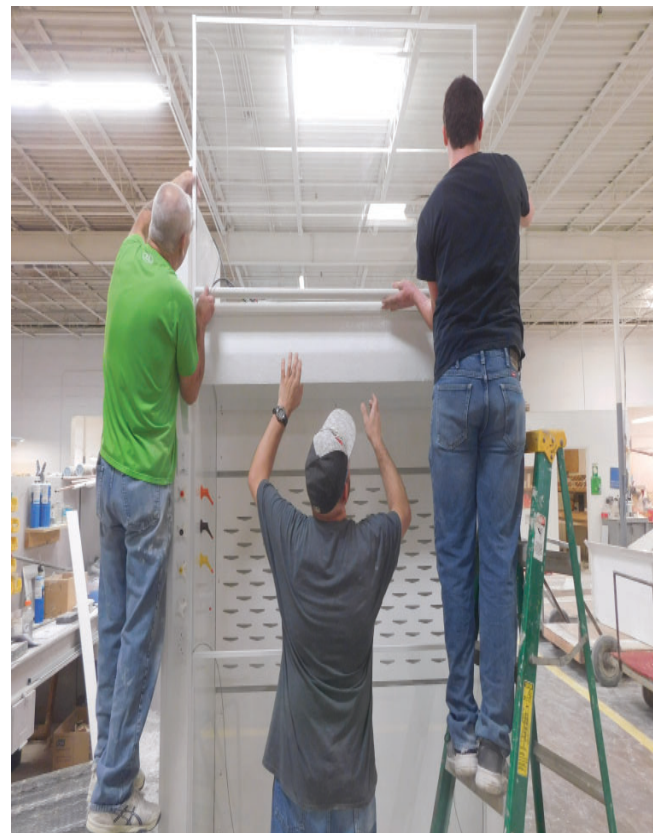
Install upper sash stop blocks from sash tracks to allow the upper sash to pass to the upper position, raise upper sash and re-install sash stop blocks.
