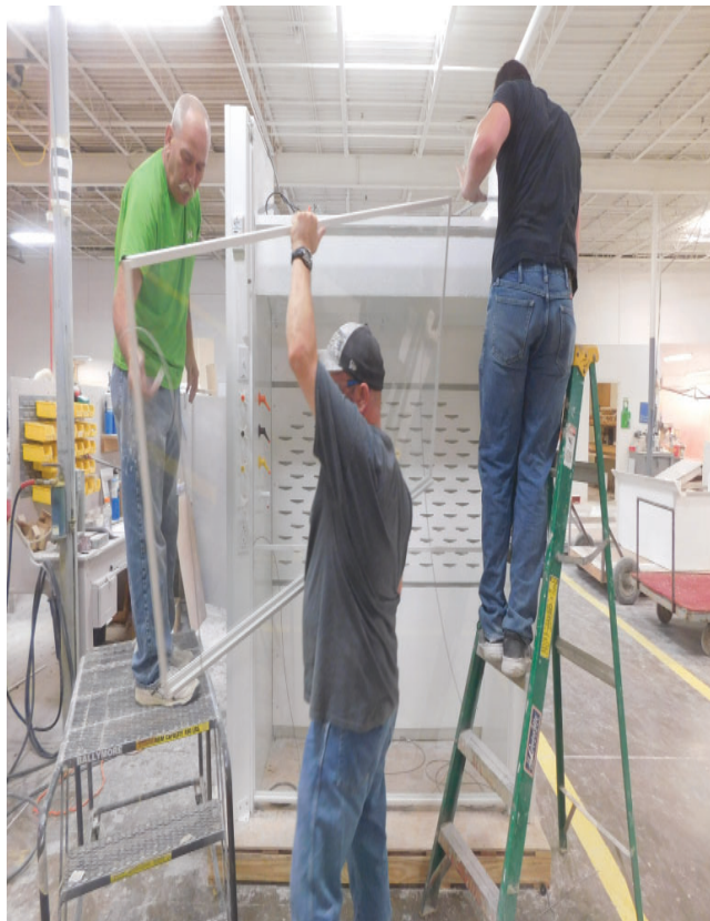
Install Lower Sash into tracks, unroll cables and insert into holes above pulleys.
