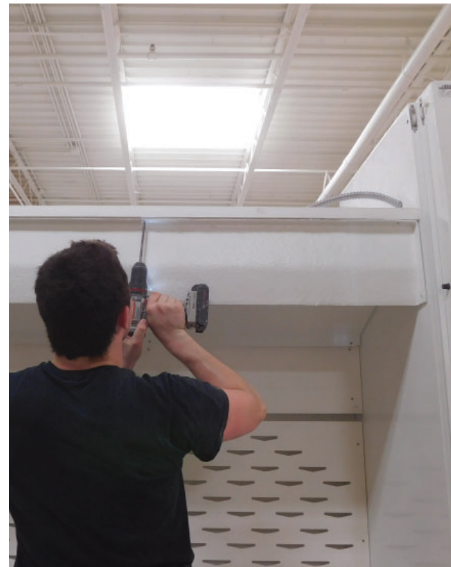
Mount Front Baffle center section to the Ceiling Panel with provided #8 or #10 sheet metal screws.
