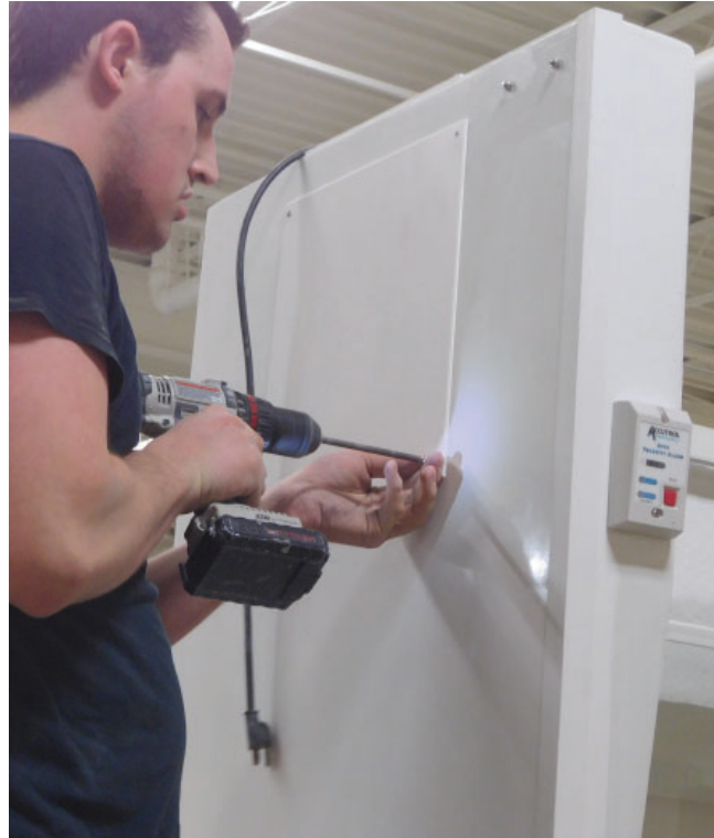
Install access panel over weight access area.
