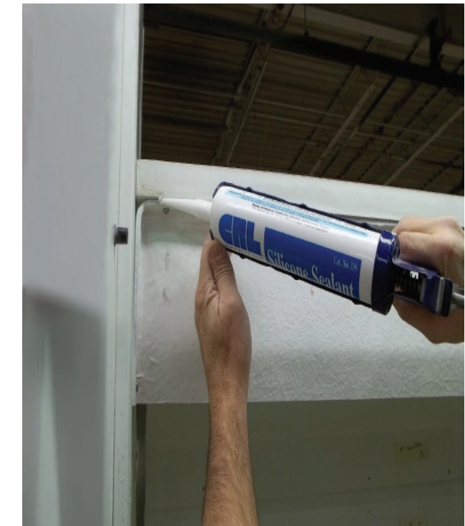
Caulk the interior perimeter of the Ceiling Panel joints with provided 100% silicone caulk.
