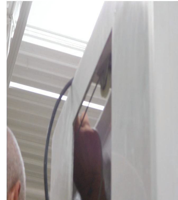
Insert the cables into holes above tracks, noting the markings directly on the sashes for orientation and location. NOTE: Finger pulls are located at the bottom of each sash.
